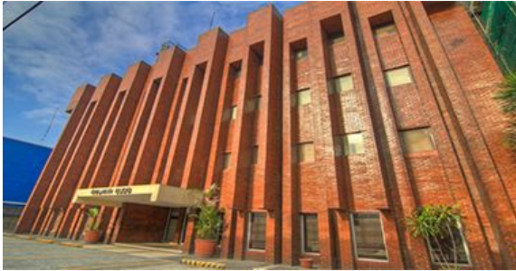
DOLMAR BUILDING EDSA
